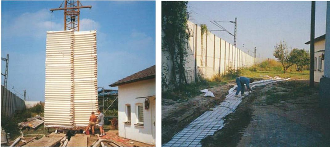
Figure 12. Installation of the gas cushion screen adjacent to a railway track in Düsseldorf, Germany, 1990. Left: installation of gas cushion screen, Right: placement of surface isolation layer.
