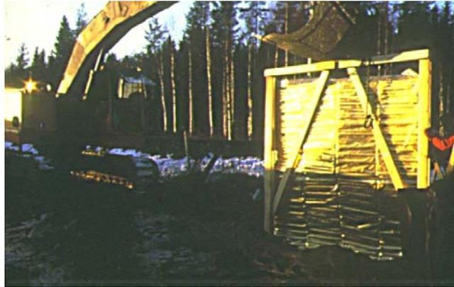
Figure 8. Installation of gas cushion screen in Bentonite slurry, using timber frame, Gnarp, Sweden 1984. First generation of gas cushion system.
